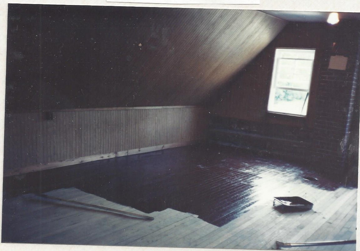
First coat of paint going on the floor upstairs.
