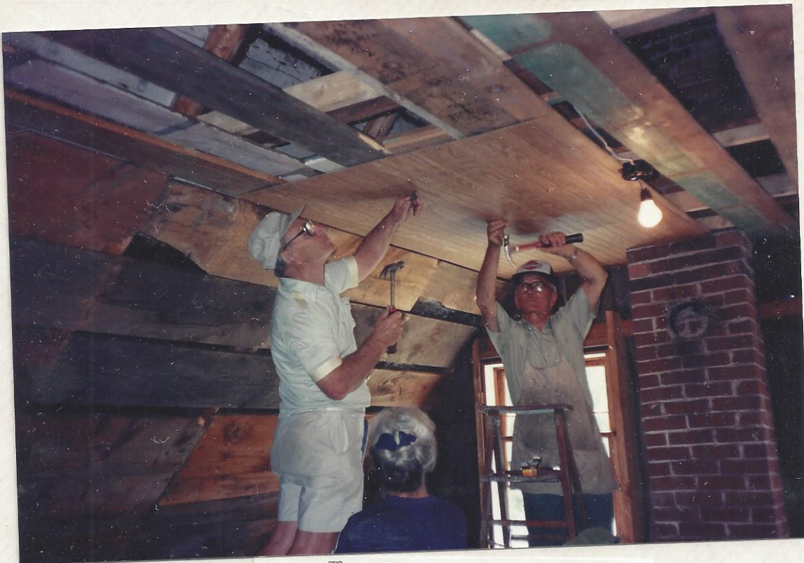
The first of the panels going up.
